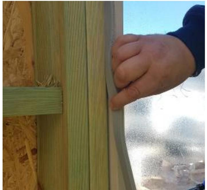
**Figure 11** Applying high density acoustic foam
