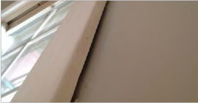
**Figure 8** An internal gap between the architrave wall.
